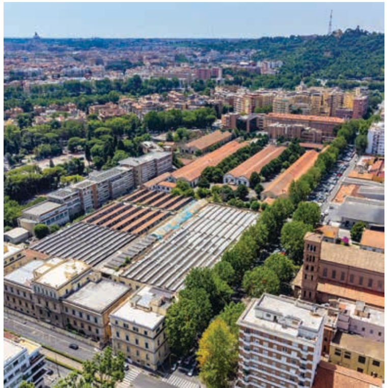
The Guido Reni army barracks in Rome, which COIMA will regenerate along with Italy’s sovereign wealth fund, CDP Group. When complete, it will be a mixed-use area that will include a new science museum.
