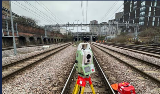
NwR tunnel investigations at York Way, Islington
