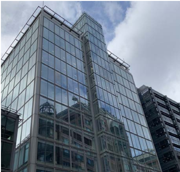
DCIF financed the BREEAM Outstanding, and Well Building Institute's platinum accredited 280 Bishopsgate
