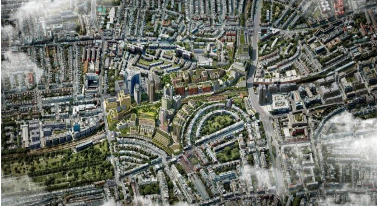
Source: Earls Court Development Company Aerial view of the 17.4ha site, looking westwards
